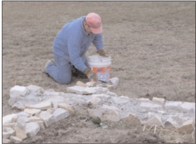
Figure 78. Cementing the ruins into place.
